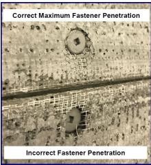
Ensure screw length selected allows for a minimum of 1" penetration into the concrete structural back-up. Calculation for minimum screw length:
