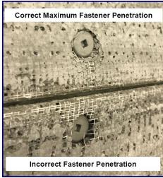
Plan view of ProGUARD DP\* and screw penetration
