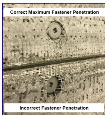
Ensure screw length selected allows for a minimum of 1" penetration into the stud structural back-up behind the sheathing. Calculation for minimum screw length:
