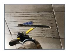
Once the ARRIS-tile unit has been cut into sections, chisel out the grout around the perimeter of the ARRIS-tile that is to be removed.
