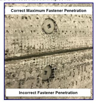
Engineer of Record should select screws and screw spacing using <u>NTA</u> <u>Report TRIG030116-28</u>. Screw spacing will be dependent on weight of the thin adhered masonry veneer or synthetic stucco application, insulation thickness, wall height, wind pressure, wind speed, and whether the installation is a **supported** or **unsupported** panel application.
