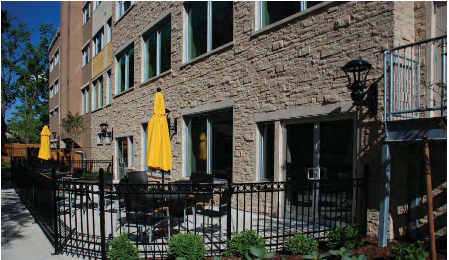
Arriscraft ARRIS-stack over ProGUARD®DP Insulated Cement Board Panels, using Laticrete MMS materials.
