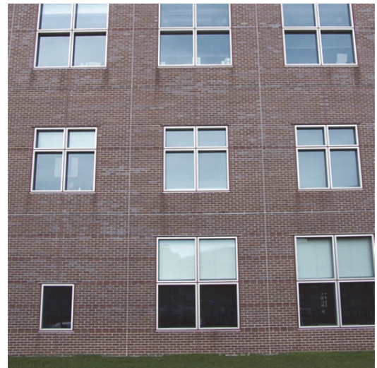
Figure 11: Placement of movement joints creates wall symmetry.
