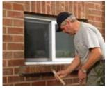
5. Tool multiple mortar joints (13 this example), and then brush excess mortar from bricks.
