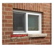
2. Insert Sill; repeat as required depending on window size (2 sills for this example.)
