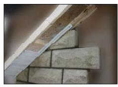
Attach J-mould to lower edge of the guide board, overlapping top edge of stone.
