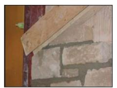
Leave a clear space of at least 1/8" between the stone and the guide board. Do not pack tight with mortar.
