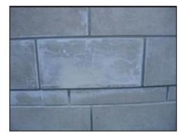
Alternatively, the use of mechanical splitter can produce a straight split with a clean front edge.
