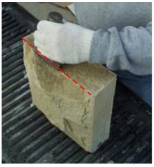
Chisel back the edges of the split surfaces to remove the excess "eyebrow" of stone. For tumbled edges, this end can be "antiqued" by light hammering of sharp edges and faces.
