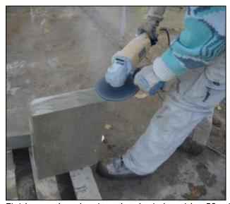
Finish smooth ends using a hand grinder with a 50-grit disk or a belt sander with 50-grit silicon carbide abrasive.
