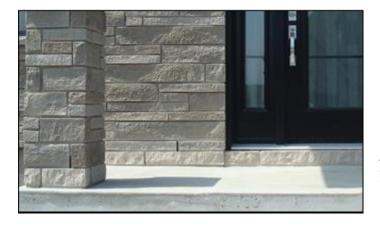
Masonry walls adjacent to porch slabs and stair treads should be built with a starter course of Adair® Limestone.
