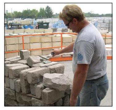
Break individual Old Mill stones into irregular shapes. Chisel back edges of broken surfaces to remove the excess "arris" of stone.
