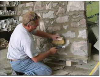
After tooling, brush excess mortar from the stone surfaces utilizing steel and soft fibre brushes.
