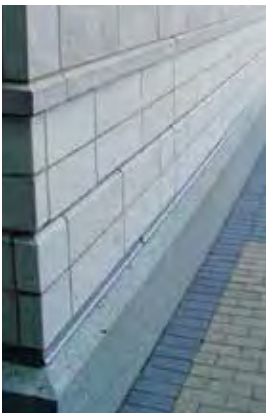
Masonry raised above grade
